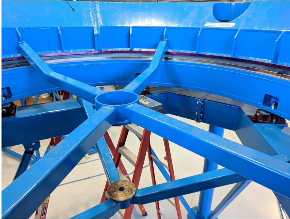
Old fixed rotary joint supports
