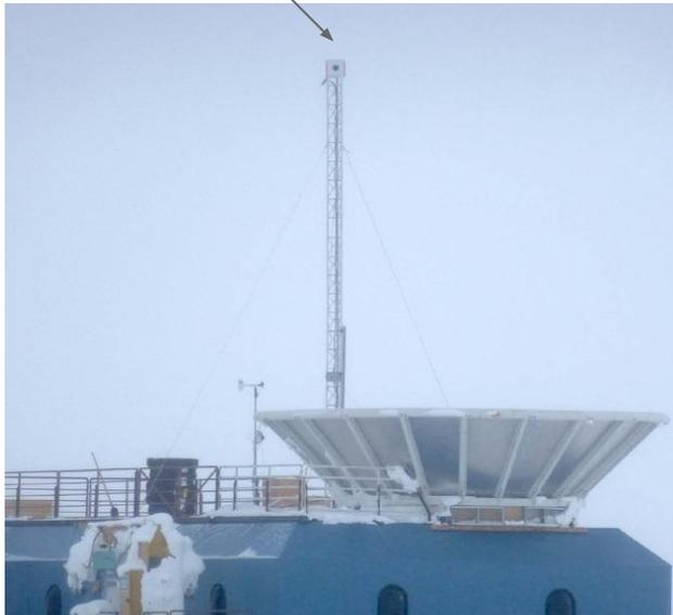
Flat mirror reflects source signal into telescope
